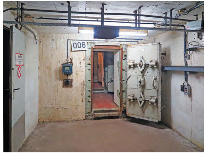
The outermost 1.6 tonne blast door at Garzau, one of four in succession. Photo Clive Penfold
